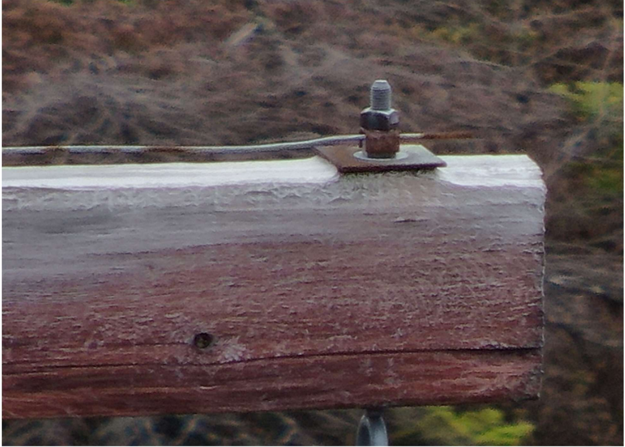
Figure B-5 – Splits through Cross Arm.
