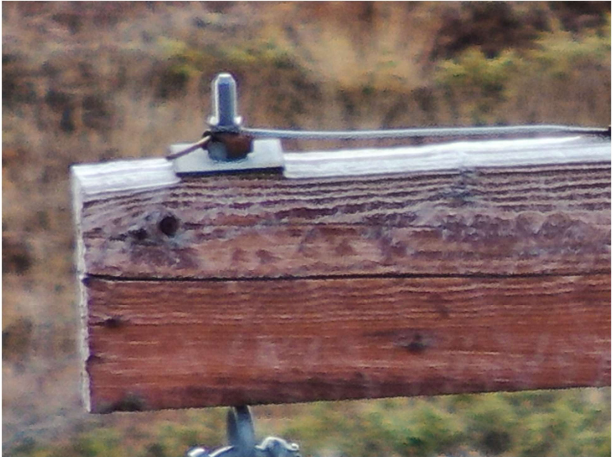
Figure B-6 – Split through Cross Arm.
